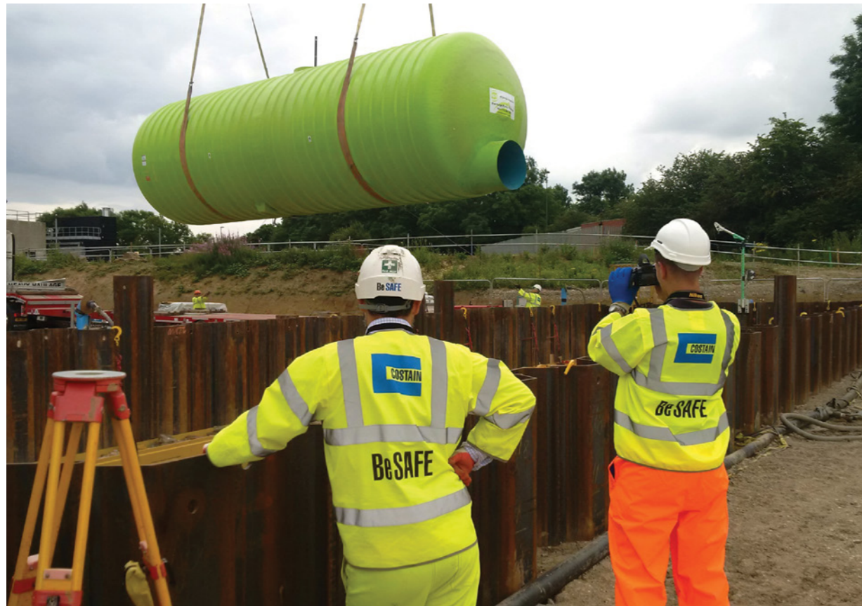
Two 170,000 litre APS Chambers being installed for the Port of Immingham
