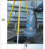
Finished access opening size is correct to tank opening size to ensure pump can be installed correctly. Finished concrete slab opening should NOT be reduced in size to that of the tank opening otherwise pumps may not fit.
