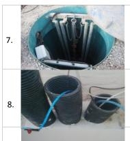
Guide brackets, galvanised steel guide rails and internal discharge pipes are fixed into tank?
